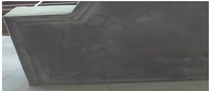
during curing. Crazing typically occurs due to environmental influences such as prolonged elevated wind speeds, high temperature or low humidity but can also occur when admixtures are improperly added to the stucco mix. Performance of stucco veneers is always dependent upon a proper plaster mixture but increased/extended curing may be required depending on ambient conditions to maintain a moist curing of the stucco.
