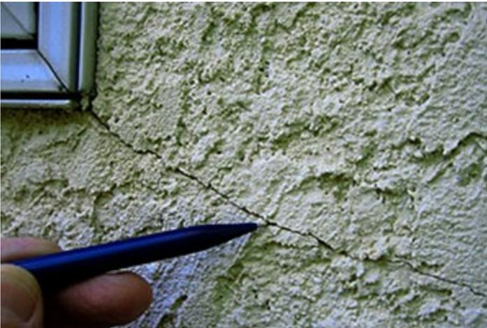
Metal framed systems are affected by many of the same stresses of wood framed systems and may also incur movement from thermal expansion and contraction. Many metal framed systems are designed for larger scale construction and the additional loads applied to the building during and/or after stucco application can cause deflection of the framing members increasing the stresses applied to the stucco.
